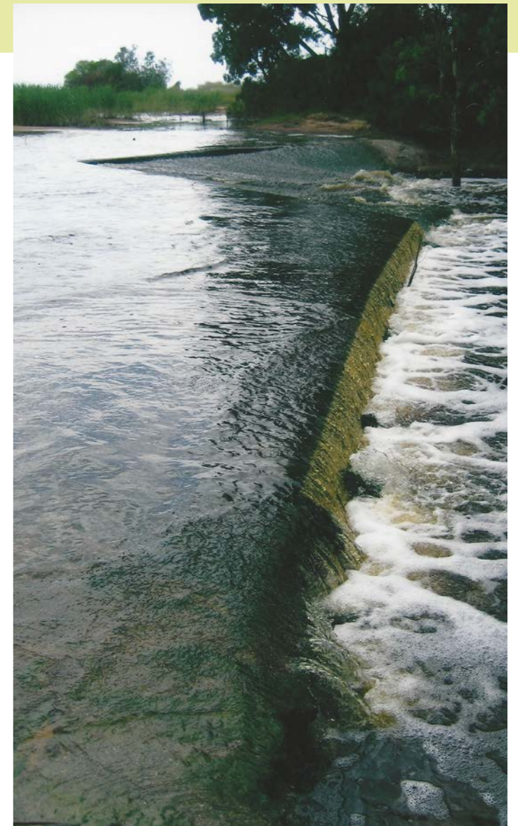
Spillway at entrance to Lake Bolac, February 2011
